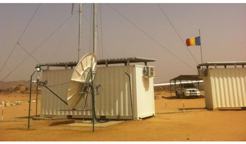
Marlink's Premium VSAT service will provide a reliable link to remotely monitor the facility in Amdjarass
