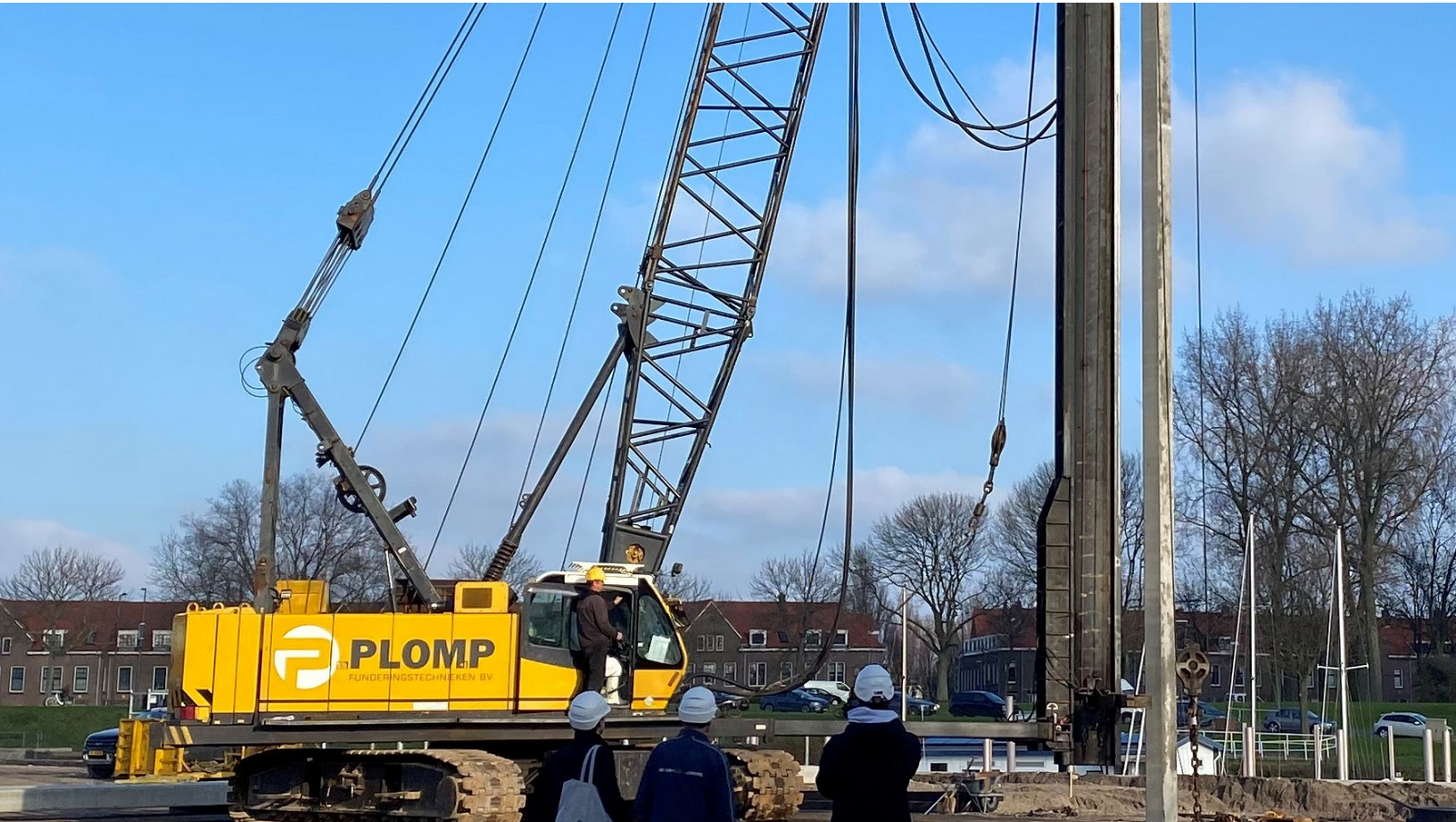
First post placed at VETUS's new 9,500m 2 facility in Schiedam, Netherlands
